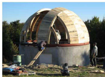
ASV observing pavilion under construction
