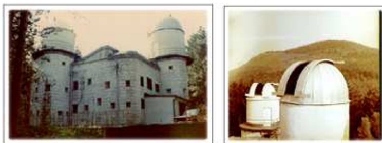
Figure 2: Old part of the observatory with two domes. In front there are foundations for a new buliding. (Middle of seventies).
