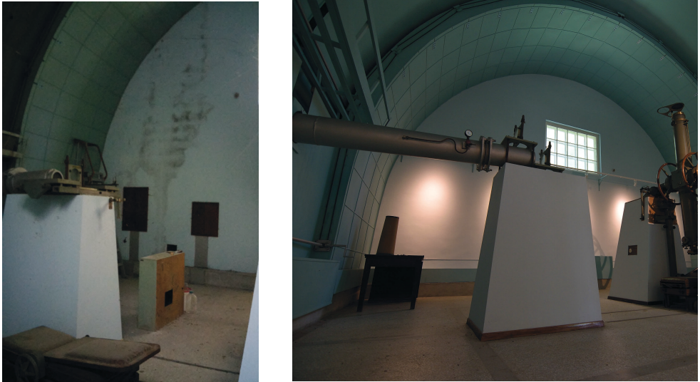
Figure 2: Photographs of the Large Transit Instrument: before remediation - left panel; after remediation - right panel.
