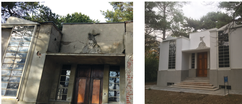
Figure 5: Photographs of the School Pavilion: before remediation - left panel; after remediation - right panel.
