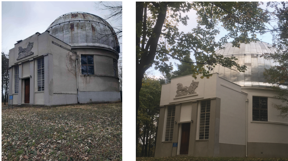
Figure 4: Photographs of the Large Refractor: before remediation - left panel; after remediation - right panel.
